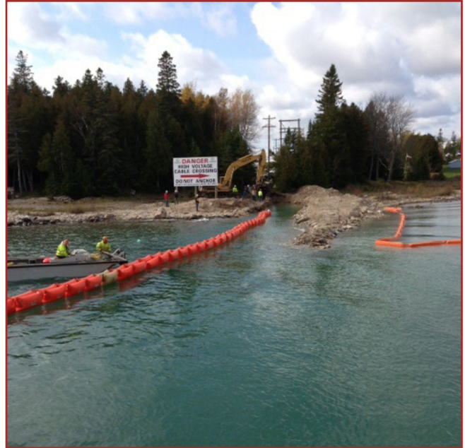
Floating the cable to shore to be terminated.
