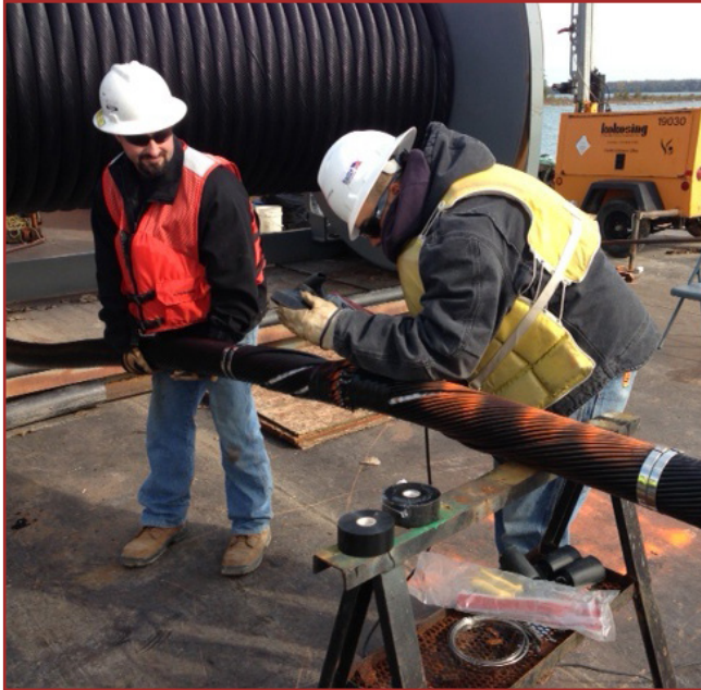
KCS Technicians cutting the armor wires back on the cable.
