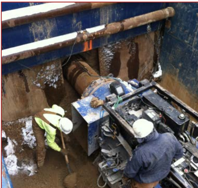
Boring under the railroad tracks.
