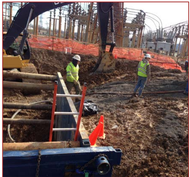
Pumping grout inside the 24" casing pipe that house the 138kV circuit.
