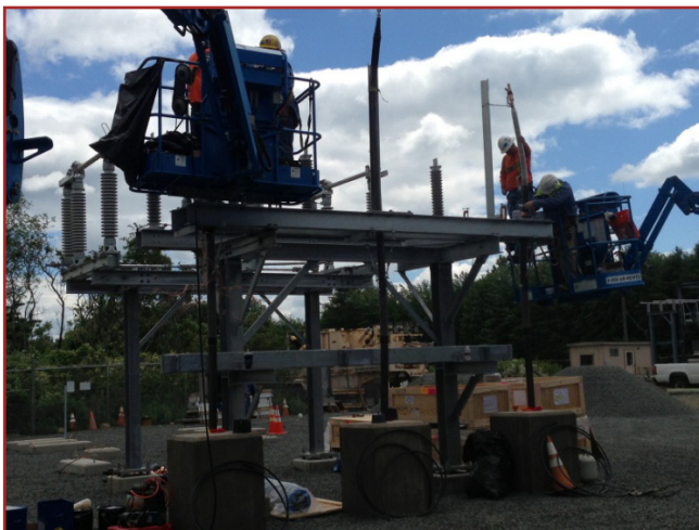
KCS Technicians securing the cable to aluminum cable stands.
