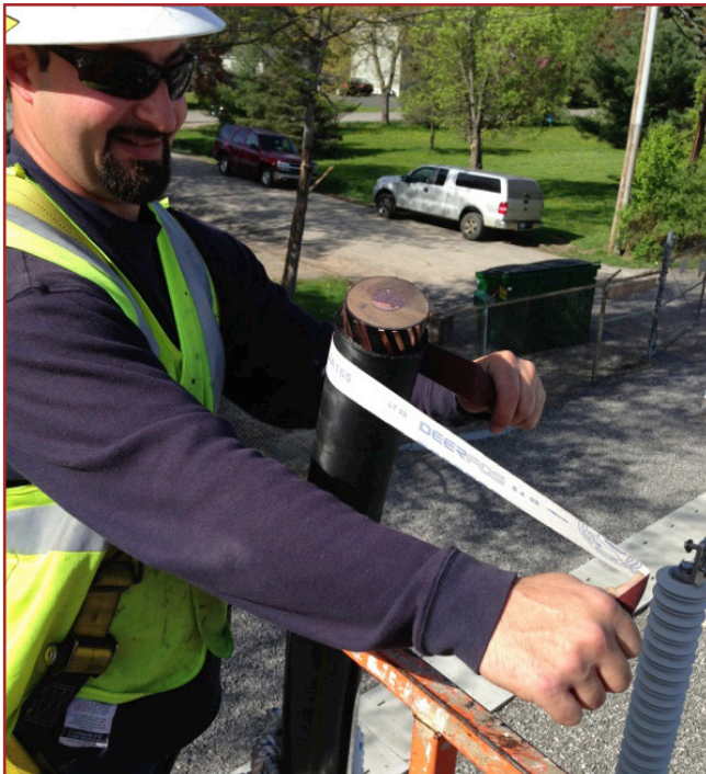
Prepping the cable for 10kV jacket test.
