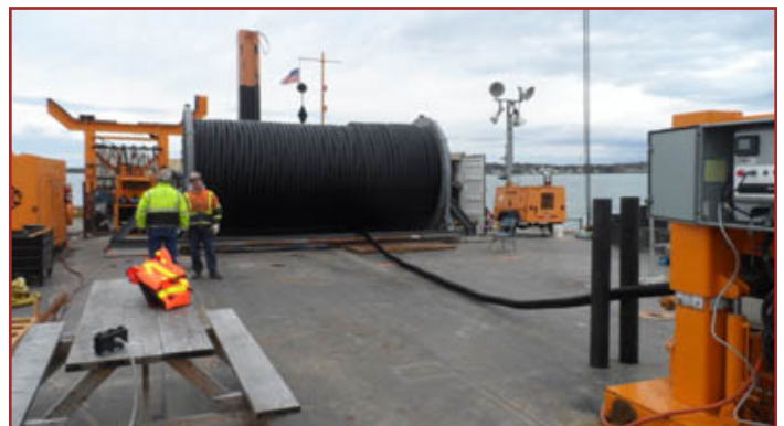
The reel is ready for the installation process
