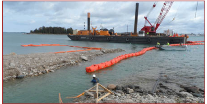
Cable floating to DeTour
